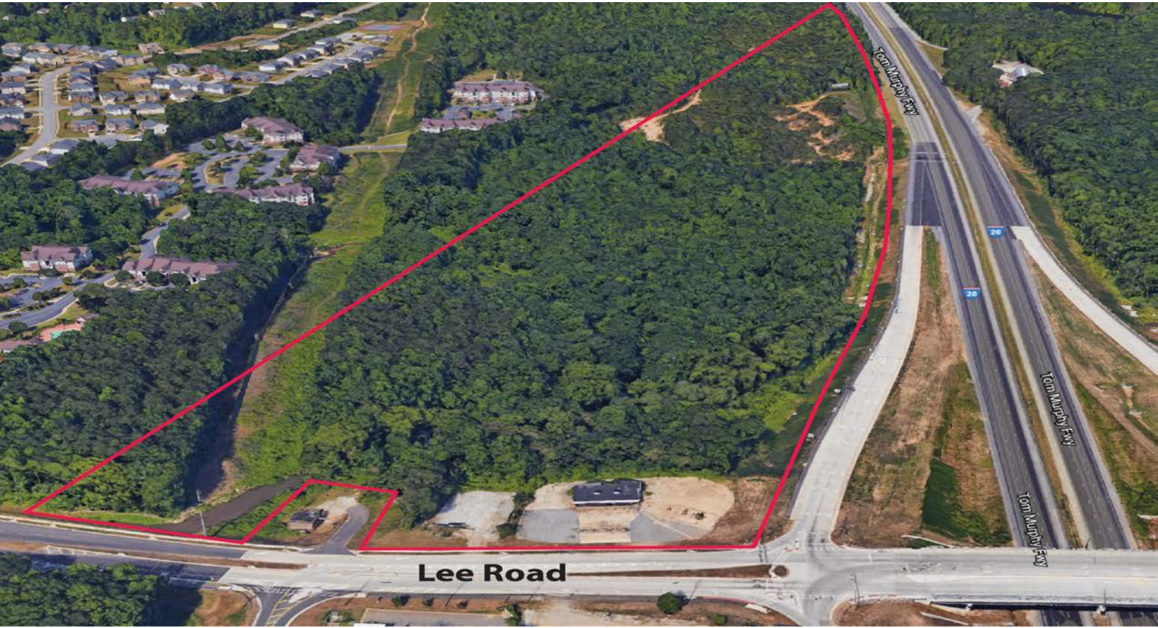
Aerial Looking West
