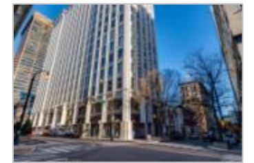
Healey Building Exterior along Walton Street
